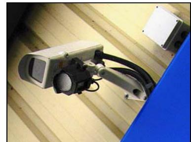
*IR-sensitive network camera with IR illuminator attached below the camera housing*
