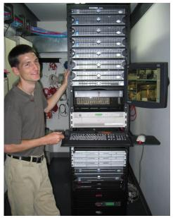
Nomad purchased an initial license for 16 cameras, but quickly expanded to 25. They are running on Windows 2000 with a dedicated Dell server and dedicated web just for the security system. Axis 2100 model cameras complete the current solution, installed at the docking bays for shipping and receiving, at the entrances and exits, reception, and internally throughout the facility in production areas, the graphics studio, and customer service.
